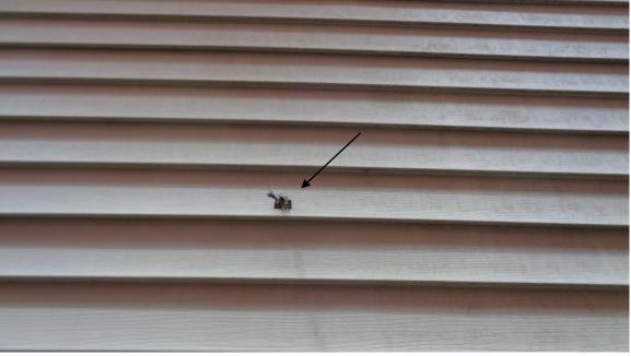
• There is a wire sticking out the right exterior wall. The wire should be eliminated or end in a junction box.
