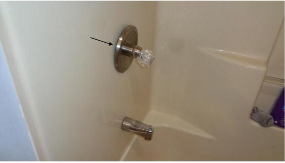
• There is a gap at the water control in the 1<sup>st</sup> floor bathroom. Water could get behind the fixture when showering.
