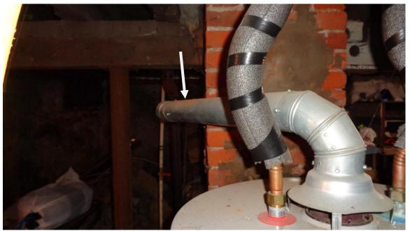
• The flue pipe on the water heater is not sloped properly. This could allow carbon monoxide to enter the house. It is important to correct this slope or install a power fan.
