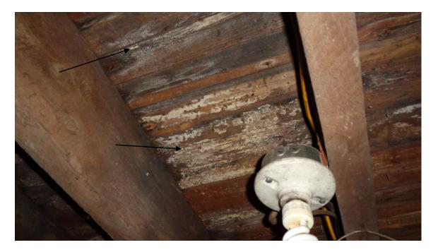
• Suspect mold growing on several floor joists and sub-floor in the basement.
