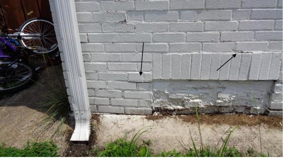
• The brick and mortar have cracked and moved under the front porch right of the steps.
