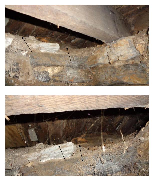
• The sill plate and rear rim joist is rotted at the rear of the basement. These area needs reinforced.
