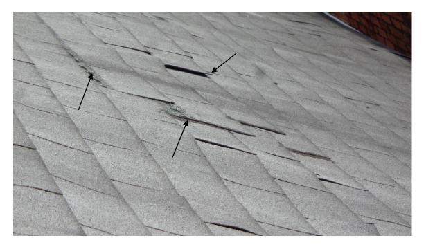
• I found 10+ shingles that are missing or loose on the main house roof. I recommend a roofing contractor evaluate and repair as needed. It is probable that the shingles need to be replaced.
