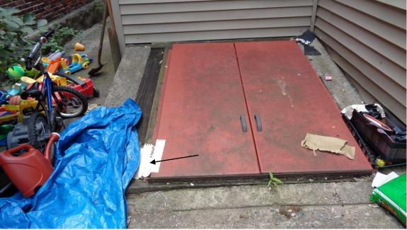
• Rotted wood that frames in the metal exterior doors to the basement.
