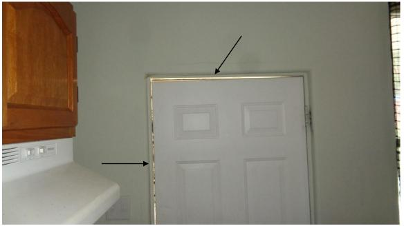
• The rear exterior door is not square in its opening. The threshold moves and the door does not close or lock properly. There is a large gap around the door when close.
