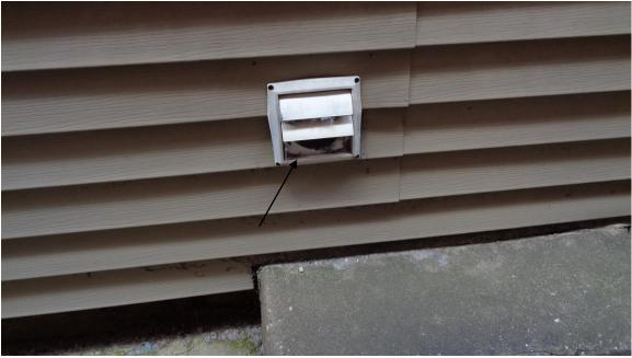
• The exterior dryer vent cover is broken.
