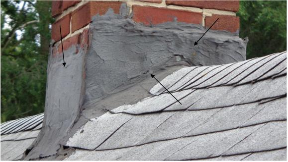
• The chimney flashing is tarred. You must maintain the tar to prevent water leakage or replace with proper flashing.
