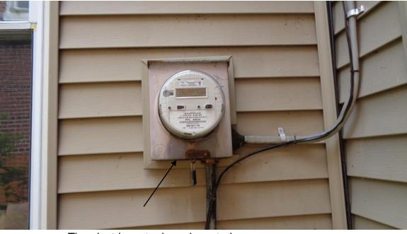
• The electric meter base is rusted.
