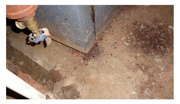
• The boiler would not turn on. There is rust around the bottom of the boiler. I recommend an HVAC contractor evaluate the heating system and repair as needed.
