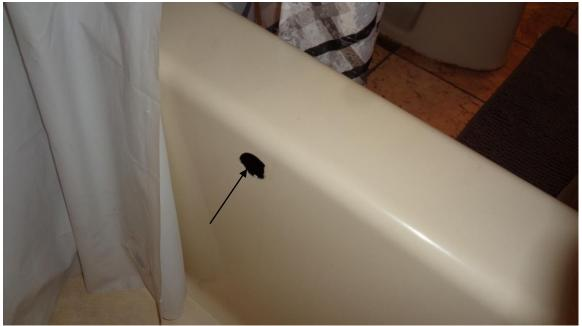
• There is a hole in the side of the bathtub in the 1<sup>st</sup> floor bathroom.
