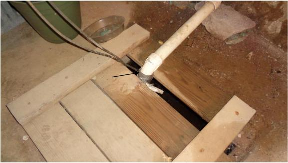
• The pipe on the sump pump is taped together.
