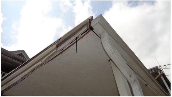
• Loose trim, gap in trim on the side of the rear rubber roof.
