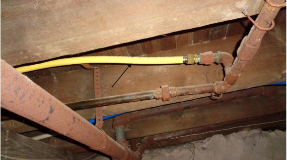
• Yellow gas flex pipe is used and I did not see a bonding strap on the steel gas pipe. The manufacture of the yellow gas flex pipe requires the steel pipe to be bonded to help prevent the pipe from bursting if lightning strikes close to the house.
