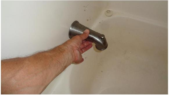
• The pipes for the tub spouts are loose in the wall. Both bathrooms.
