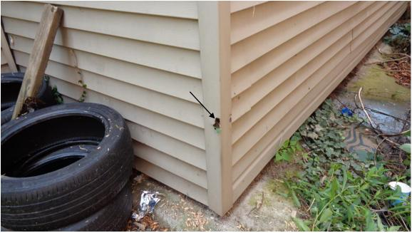
• Minor siding damage on the left rear corner of the house.
