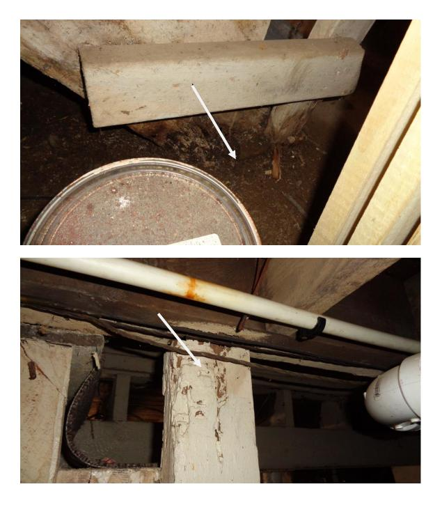
• Rotted/termite damage wood support and rotted/termite damage stringers on the basement steps. The steps should be repaired.
