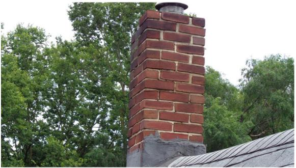
• Loose brick and mortar on the chimney. I recommend a mason evaluate and repair as needed.
