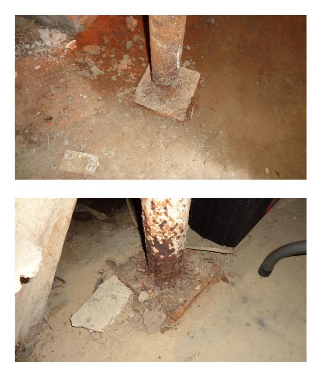
• The bottom of the metal support posts are rusted in the basement. These posts need painted to prevent further rust.
