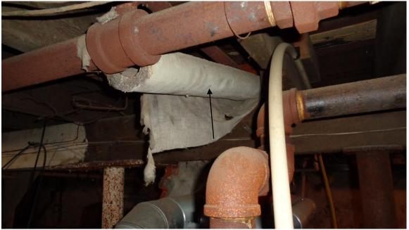
• The white insulation on some of the heat pipes in the basement may contain asbestos.
