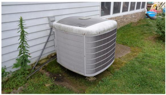
The air conditioner operated from the thermostat and provided cool air. Temperature differential of about 20 degrees which is good. MFD: 2013. Service yearly.
