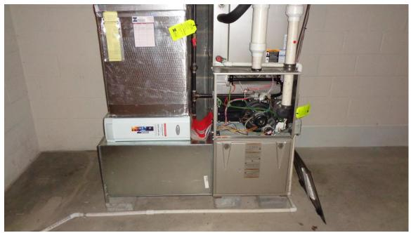
The furnace operated from the thermostat and provided warm air. Heat rise was within manufactures specifications. MFD: 2013. Service yearly.
