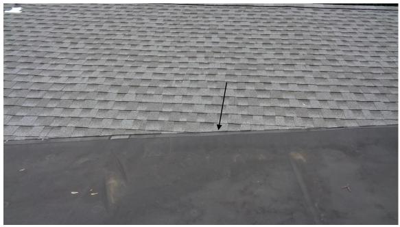
There are stains in the ceiling in the sunroom. This appears to be from water leaking where the rubber roof intersects the shingles. I recommend the shingles be lifted in this area to see how the rubber roof is sealed.
