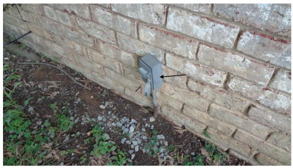
No power and loose receptacle on the left exterior wall.
