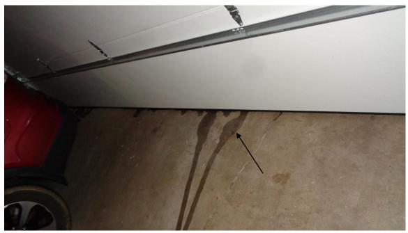
Water leaking in under the garage door when it rains hard.
