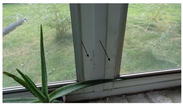
The sunroom is a manufactured room. The panels that hold the windows are made of wood that have a laminated finish. The finish is pitted and starting to delaminate. The wood inside is starting to deteriorate. Caulking the seams will slow down the rot process. Budget to replace.
