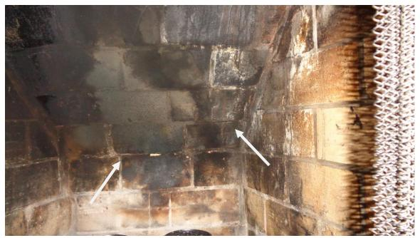
• Gaps in the mortar between the brick in the fireplace burn chamber. The gaps should be filled with mortar before used.
