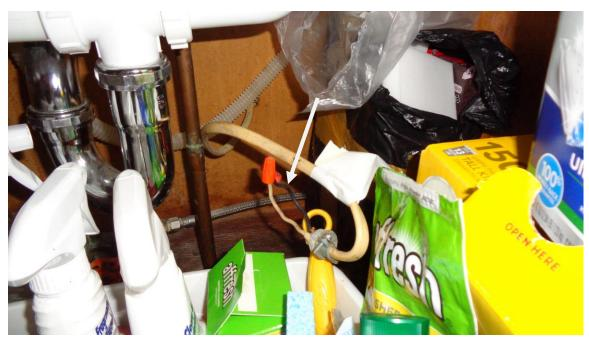
There is a wire under the kitchen sink for a garbage disposal. The wire only ends with a wire nut. The wire should end in a junction box.
