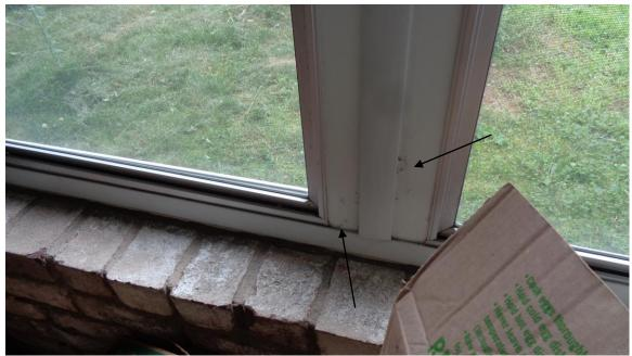
The sunroom is a manufactured room. The panels that hold the windows are made of wood that have a laminated finish. The finish is pitted and starting to delaminate. The wood inside is starting to deteriorate. Caulking the seams will slow down the rot process. Budget to replace.
