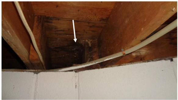
Rotted wood under the exterior door out of the laundry room. This
