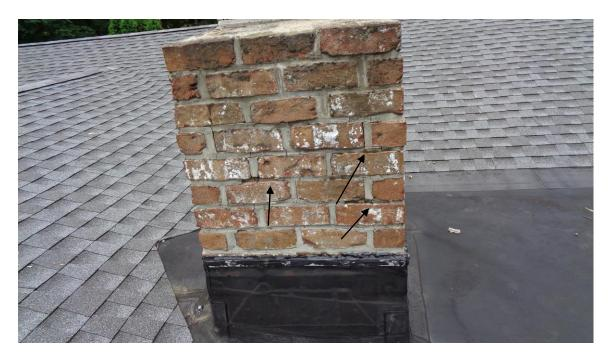
Cracks and gaps in the mortar between a few of the brick on the chimney. The chimney needs pointed.
