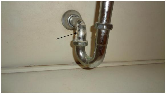
The bathroom sink traps are pitted under most of the sinks.
