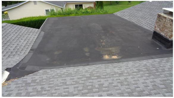
• The rubber roof material is in good condition.
